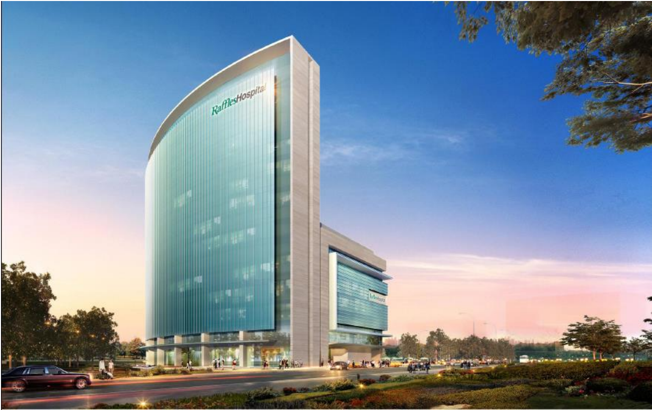
Image 1: The Shanghai New Bund International Hospital Project
